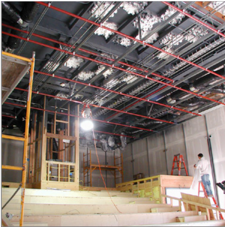
The theatre under construction, summer 2004.
