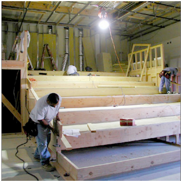
Building the riser. Note all wood construction.
